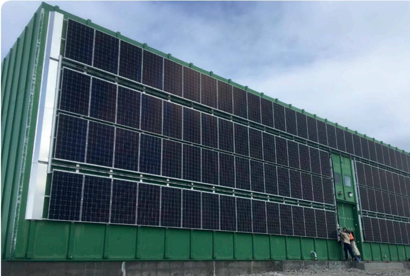
**Above:** The 105 solar panels were installed with a wind deflector to minimise the effects of high wind speeds during blizzards
